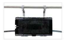
16. Attach the closure to the mounting rod. Complete the installation.
