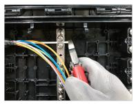
7. Place the strength member under the strength member retention plate. Fasten the strength member retention bolt and retain the strength member.
